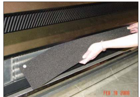
Figure C: Remove Filter Media
