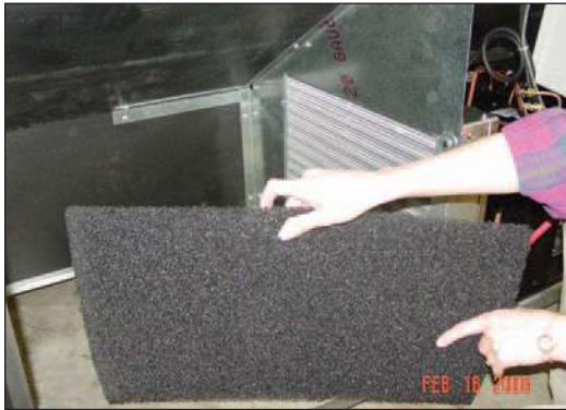
Figure B: Filter Media Removal
