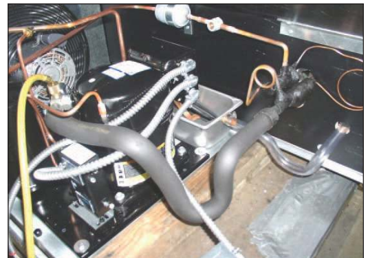
Figure C: Drain P-Trap Tubing
